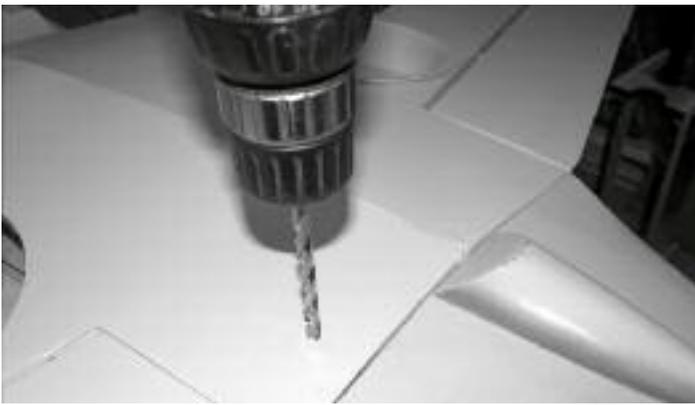
29. Drill a 1/4" hole through the wing and wing mounting plate at the marks made in the previous step. Insure the drill is straight and the wing is aligned and held securely in place.
